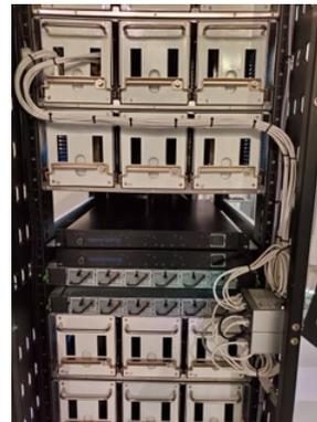
**Photos:** Natron BlueTray4000 batteries deployed in a Forced Physics platform at H5 Data Centers' Phoenix facility.
